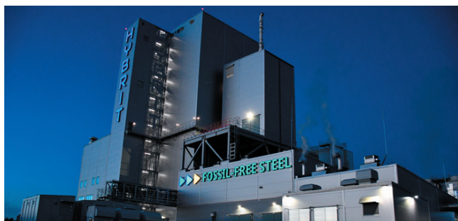
HYBRIT direct reduction pilot plant, Luleå
